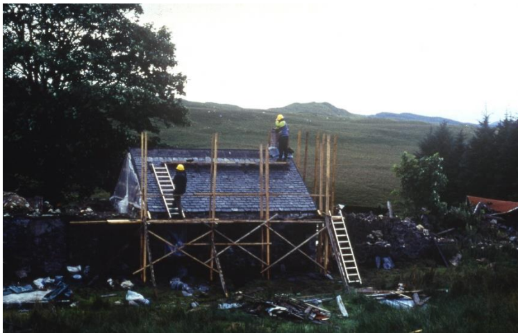
Slating work well-progressed
