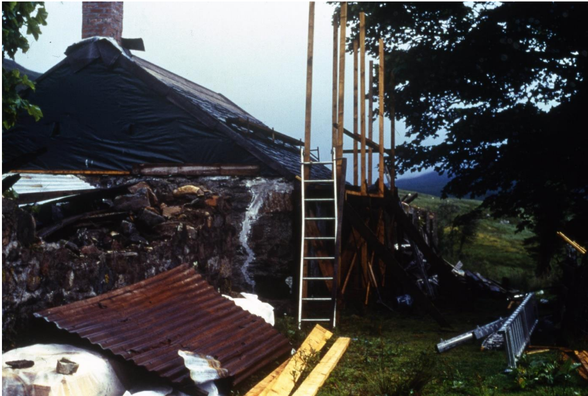
A clutter of materials as the work progresses
